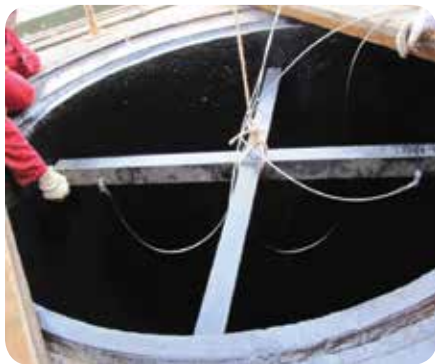
FIGURE 3 Steel frame setup for suspending Inhibitor B pouches.
