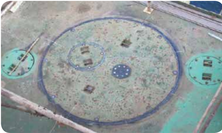
FIGURE 5 Caisson leg sealed cover.
