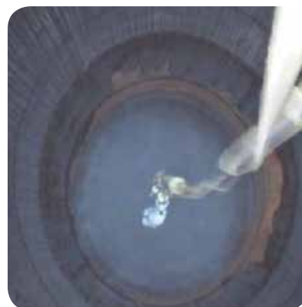
FIGURE 2 Application of Inhibitor A using a pipe coater.
